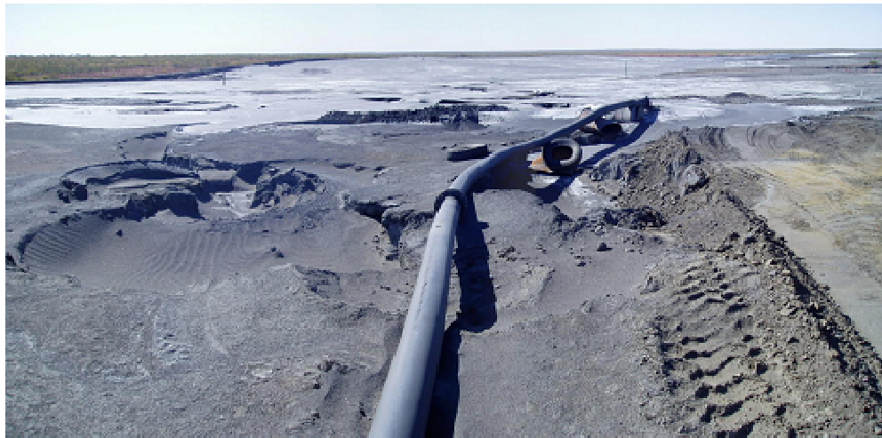
Figure 10: Typical delivery point showing HDPE pipe issues
