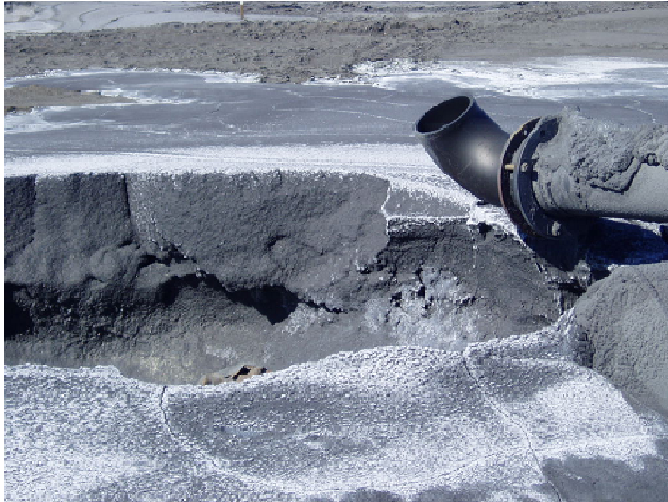
Figure 8: Photograph showing the “up-turned” pipe discharge
