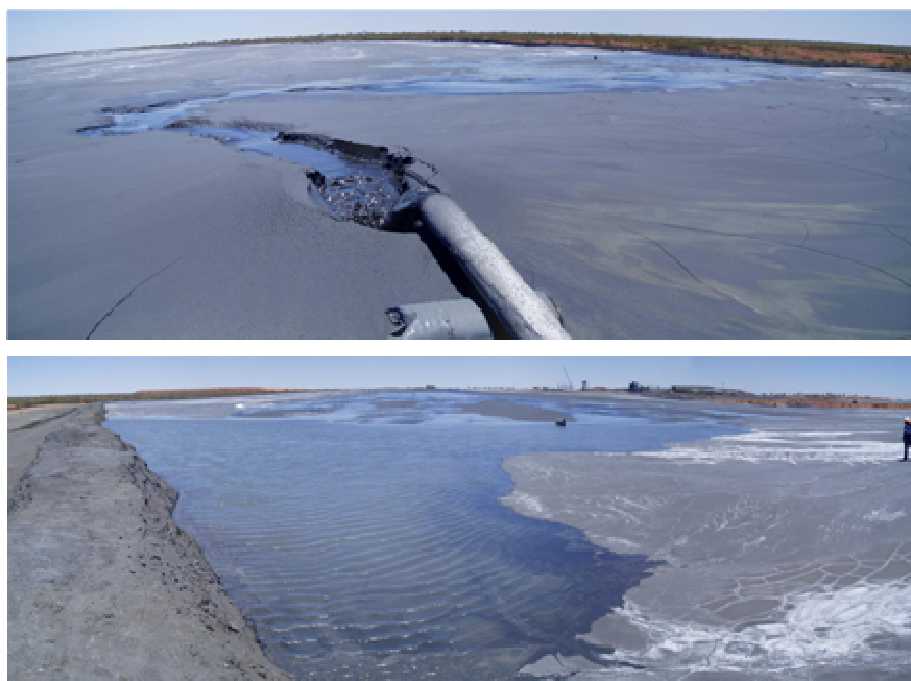
Figure 9: Ponding against the toe wall at the intersection of two advancing cones
