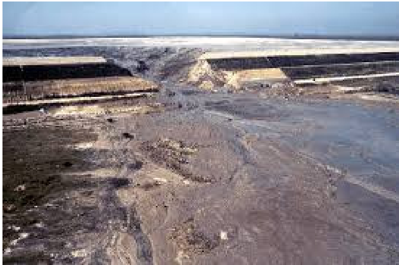
Figure 10: View of the Merriespruit flow slide close to the crater
